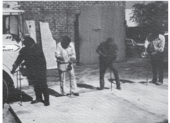
Raising Test Slab 4.
