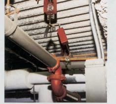
The clevis hanger in the center of the photograph fell apart and the rear hanger clevis is sufficiently displaced to have bent the ceiling bolt. There are chatter marks on the pipe in the front clevis, all indicating that this system went into resonance even though the accelerations were only 0.15gV and 0.2gH. Proper sway bracing, axial restraint and upper limit stops could have prevented this damage.
