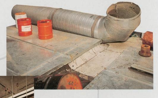
Duct work is very susceptible to seismic damage. Notice the straps that held the ducting that is now on the floor shown in Photograph to the left. This can be prevented by the use of sway bracing to limit sway and keep the duct work in place. Input was 0.15gV and 0.2gH.
