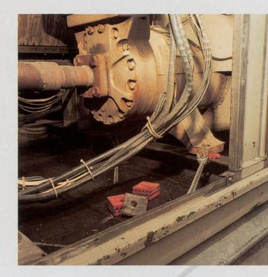
The cable system is an emergency measure to try to keep the compressor in place in anticipation of after shock. Forces were small at approximately 0.15gV and 0.2gH. Equipment with hard mounted internal components and external cushioned seismic isolation systems have a better chance of remaining operative.
