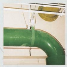
A typical example showing the use of a cable sway brace with swivel fittings for the specific purpose. Fittings are adjustable and the installation simplified by their use. (Mason Type SCB)
