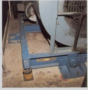
This large fan did not come down because there were control cables to prevent pendulum motion. Unchecked swaying bends suspension rods and can ultimately cause failure allowing the unit to break free and fall as in the photoghraph below.
