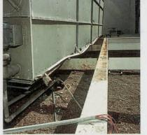
The independent rails rotated around their longitudinal axis, snapping anchor bolts and bending the cooling tower base. The problem could have been prevented by using a one piece structural base and double acting snubbers.
