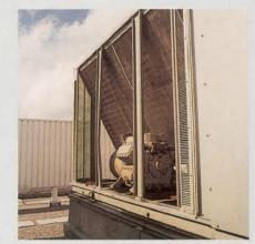
Building codes are not concerned with internal mounting systems as the codes are meant for life safety rather than contained equipment disruption. Internal components are subjected to severe damage as are external systems if they do not have proper seismic snubbing devices. Internal damage can be more expensive and harder to repair than external. Typical problems are torn up bearings, couplings, fittings, coil damage, etc.
