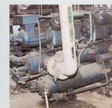
Another example of gray iron mounting failure. Fragments shown in the lower left and lower righthand corners can be dangerous to building personnel as well as equipment. Not only is the compressor out of service, but there is the additional worry of potential liability and damage.
