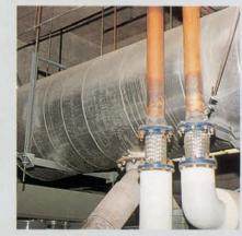
The metal flexible hose prevented pipe failure. However, the metal hose on the right was compressed. Braided metal hoses cannot accept compression and it had to be replaced. Flexible metal joints do not have the same movement capabilities as rubber joints, and tend to fail under seismic conditions. The seismic input was 0.15gV and 0.2gH. (Recommendation: Mason Safeflex SFDEJ)
