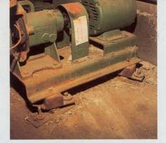
Mounting a pump directly on mountings without a supplementary steel or concrete base is bad practice because of pump coupling alignment problems when torque twists the bases. The mounting housings proved inadequate as the vertical restraining bolts failed. The restraining angles bent and either the anchor bolts were sized inadequately, of the wrong type or poorly installed as the anchorage broke free and the pump shifted out of position. Input was a low 0.2gV and 0.25gH.
