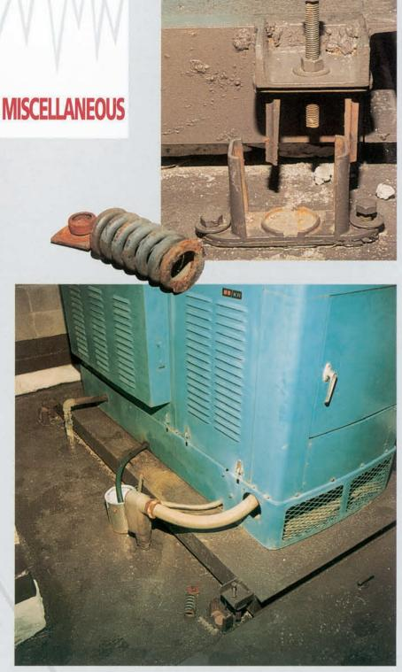
The duct work and piping in this photograph is almost all supported by spring hangers. However, the cable sway bracing kept everything in place and there were no failures in this area.
