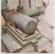
Another example showing free standing springs cannot be used without snubbing devices. The anchor bolts under these spring mountings were too close to the edge, and broke the housekeeping pad. Forces were relatively low at 0.2gV and 0.25gH, but more than sufficient to create havoc on this unsnubbed, resonant system.
