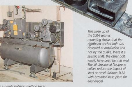
This is a simple isolation method for a horizontal tank mounted compressor (if the base legs are sturdy enough) without the use of a supplementary steel base. Mountings have built in seismic snubbers with ratings from OSHPD in the State of California. Not only these mountings, but similar designs were successful in every reviewed location. Forces were approximately 0.2gV and 9.25gH. (Mason SLRA Mountings)
