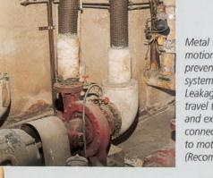
Metal flexible hose is designed to accept motion at right angles to the axis. The hoses prevented pump body failures, but after the system was back on line, the hoses leaked. Leakage was caused by metal fatigue, over travel transverse to the axis or compression and extension. Double sphere rubber connectors are all directional and can respond to motion in any direction without failure. (Recommendation: Mason Safeflex SFDEJ)
