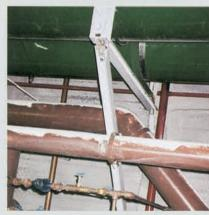
The swivel sway brace fittings at the ends of the angle iron brace eliminate welding, fitting and fabrication time. Solid sway braces can only be used on equipment that is not isolated. When equipment is isolated, bracing must be by cable or isolated devices to prevent transmission of vibration. (Mason SSB)
