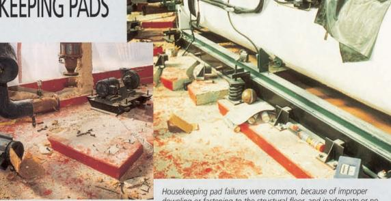
doweling or fastening to the structural floor, and inadequate or no reinforcement in the pad itself. These pads, as the pads on the cover, had both problems. Inadequate fastening allows the pads to lift, chatter and shift. Poor reinforcement allows breakage. When the pads fail, the system must fail as nothing remains in place.
