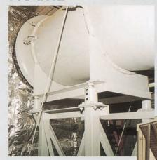
This excellent design uses square steel tubing as the support columns, cross braced by steel angles. The frame was securely fastened to the structure and the isolation positioned on top. Self-contained ductile iron, seismic mountings supported a supplementary steel base under the blower. The system was subjected to very high forces of 1.4gV and 1.2gH with no failure to the system. (Mason Industries' MS Lower Base, SSLFH Ductile Iron Seismic Mountings, MSL Steel Base)
